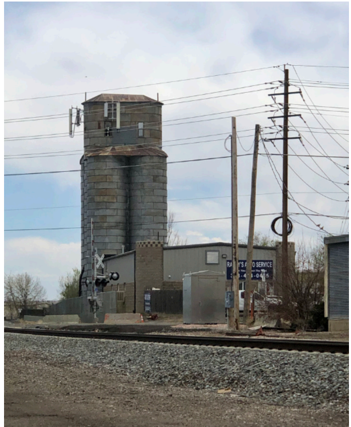
Grain elevator, Colorado Milling & Elevator Company. Location: Intersection of Colman's Way and West 120th Avenue.
